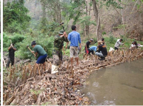
Pictures of the joint maintenance and reinforcing of the weirs of the Pşa Kényau local wisdom every year.
