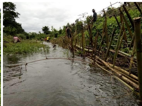
Picture of using wood and planting chrysanthemum, Ton Khrai Nam, local plants along the banks of the Pam River. to help prevent river bank erosion
