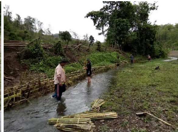
Pictures of the joint maintenance and reinforcing of the weirs of the Pşa Kényau local wisdom every year.
