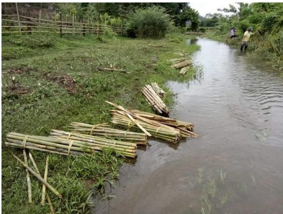
Pictures of the use of wood and the planting of the chrysanthemum, Ton Khrai Nam, a local plant along the bank of the Pam River. to help prevent river bank erosion
