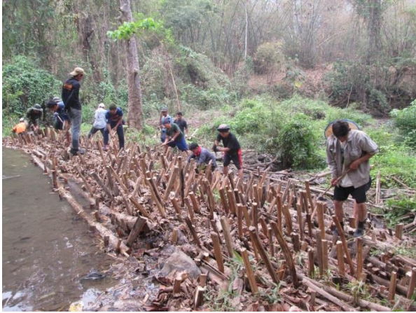
Pictures of the joint maintenance and reinforcing of the weirs of the Pşa Kényau local wisdom every year.
