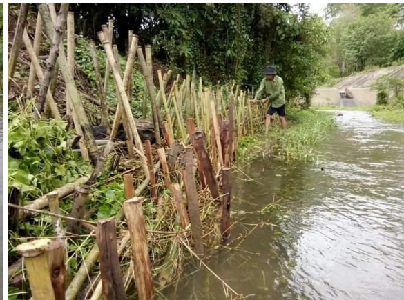
Pictures of the use of wood and the planting of the chrysanthemum, Ton Khrai Nam, a local plant along the bank of the Pam River. to help prevent river bank erosion
