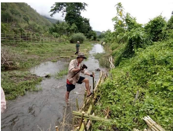
Picture of using wood and planting chrysanthemum, Ton Khrai Nam, local plants along the banks of the Pam River. to help prevent river bank erosion
